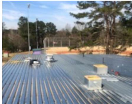
*Figure 2 S. Atl – Mechanical Roof Curbs*
